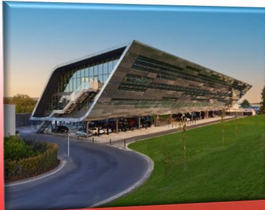
Neubau Flagship Store Herford
